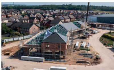
Site progress of the new Co-op store at Wynyard Park
